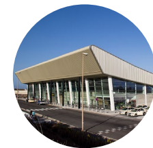
Praia Nelson Mandela International Airport (IATA: RAI)
